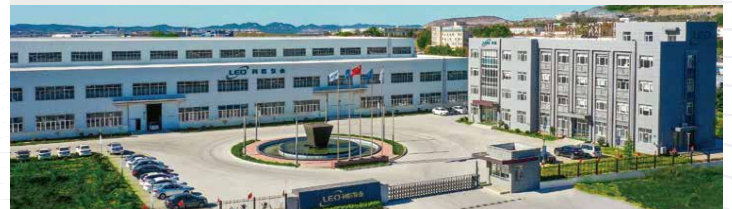
Pump Manufacturing Base for Petrochemical Industry
